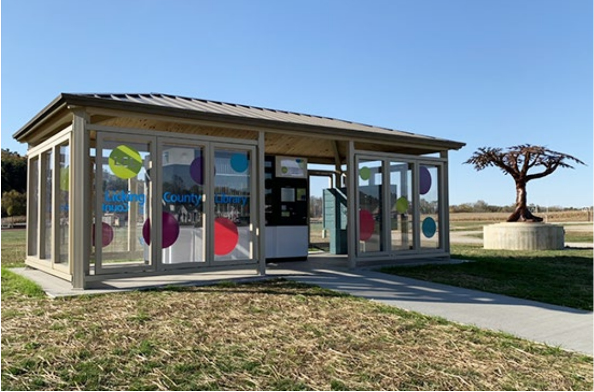
Image 43 - Library Kiosk in Legacy Park
