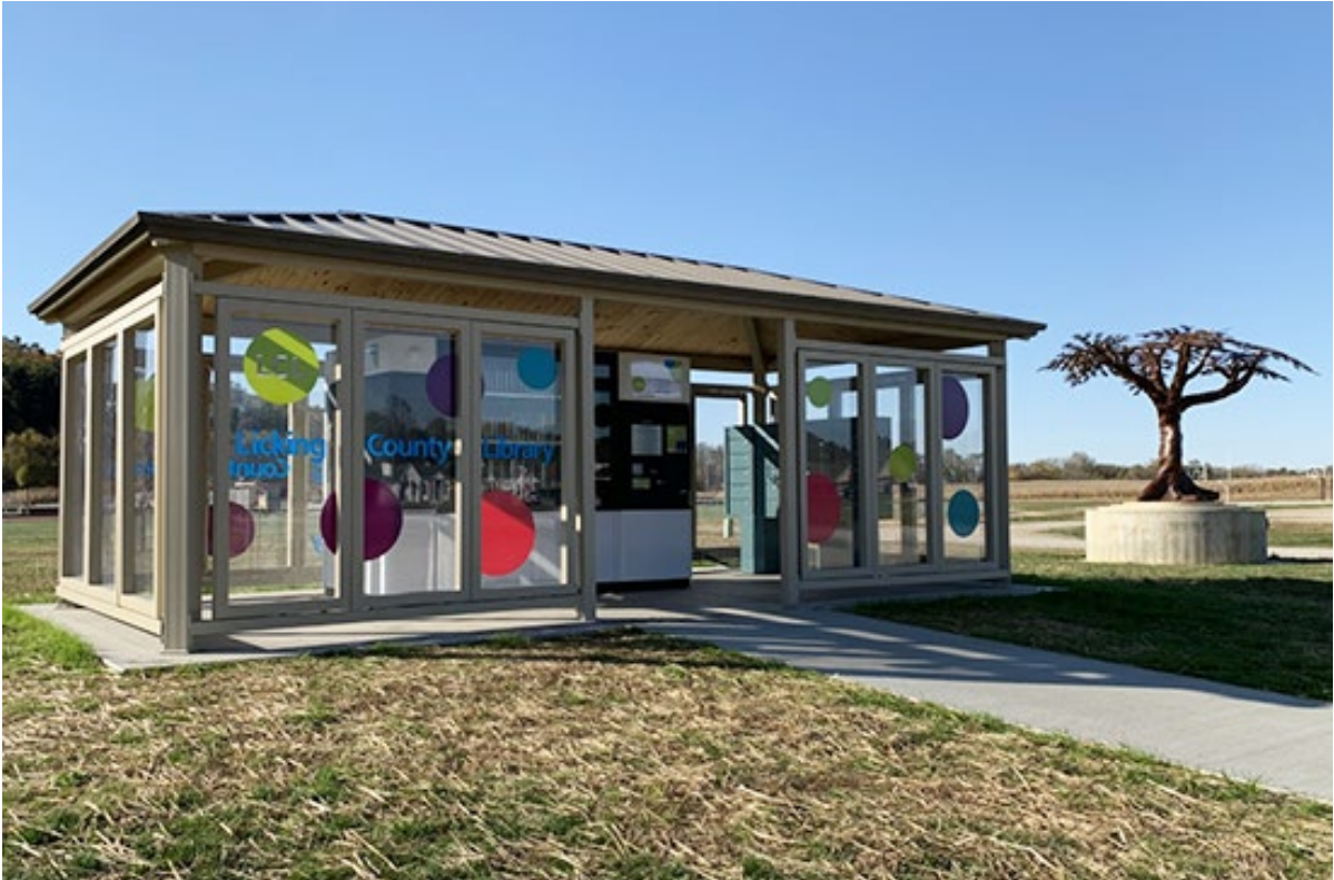
Image 44 - Library Kiosk in Legacy Park
